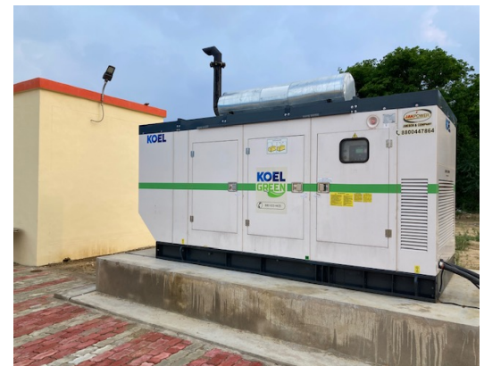
Genset with acoustic Enclosure West Campus
